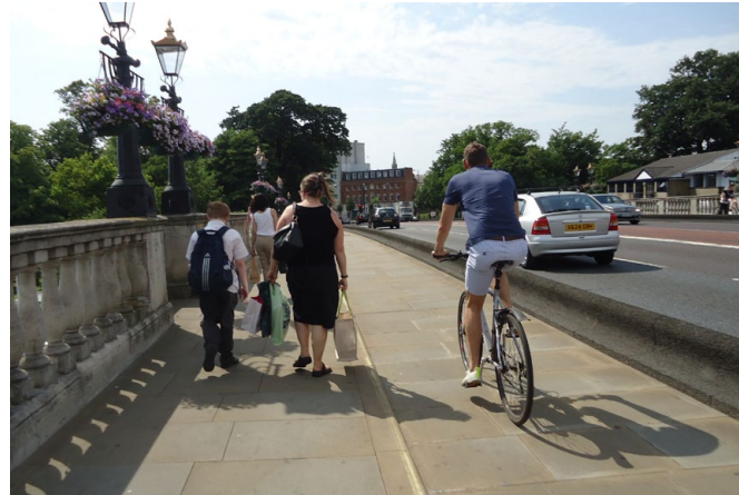
Example of a segregated cycleway on a bridge
