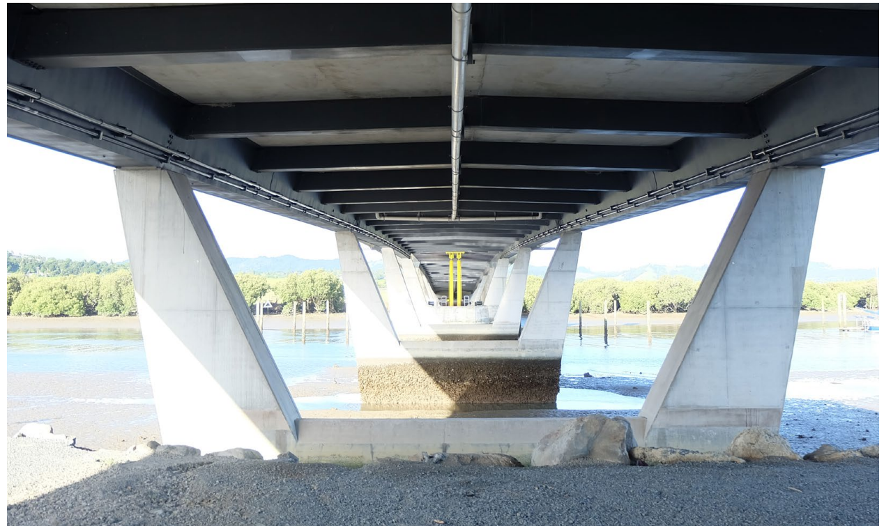
Example of good pier design - Lower Hatea Crossing, New Zealand
