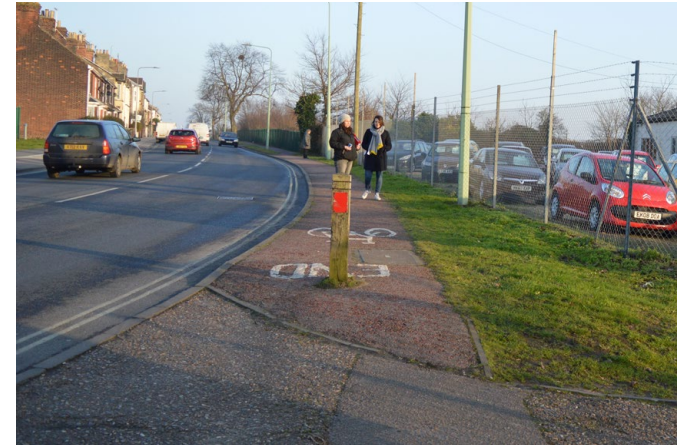
Example of a poor cycle facility with no footway
