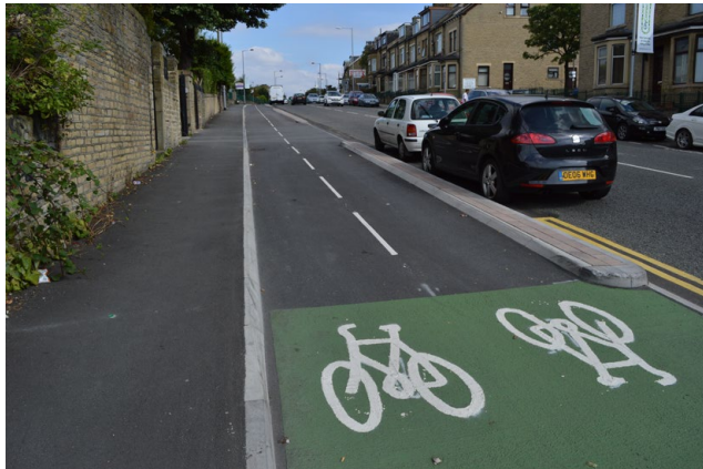
Example of segregated footway and cycleway
