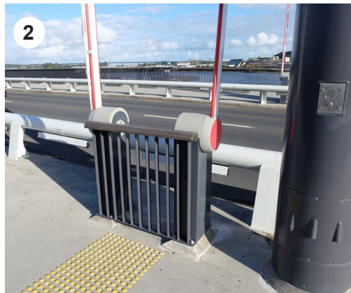
Example of wigwag and barrier system on a bridge
